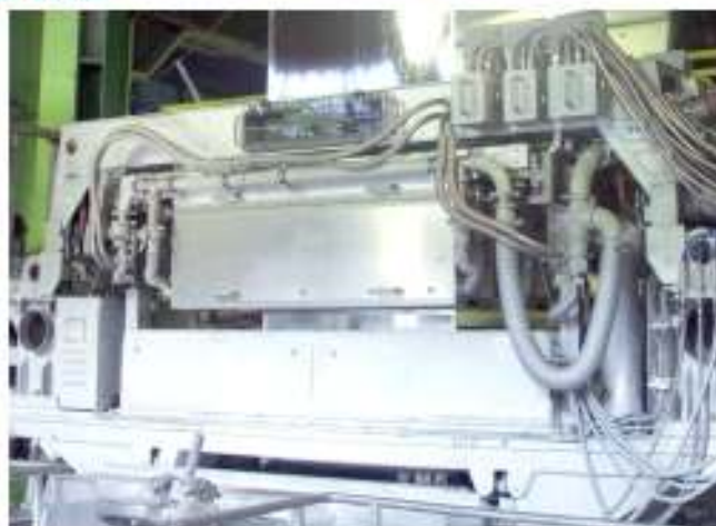
Fig.2: eMASS at the hot-dip galvanizing line FBA1 at ThyssenKrupp Steel AG in Duisburg, Germany
