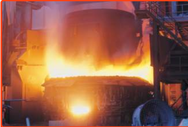
Electric Arc Furnace at Essar's Steel Plant at Hazira, India
